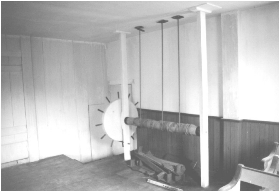
Partition mechanism at Sandwich Meeting House
