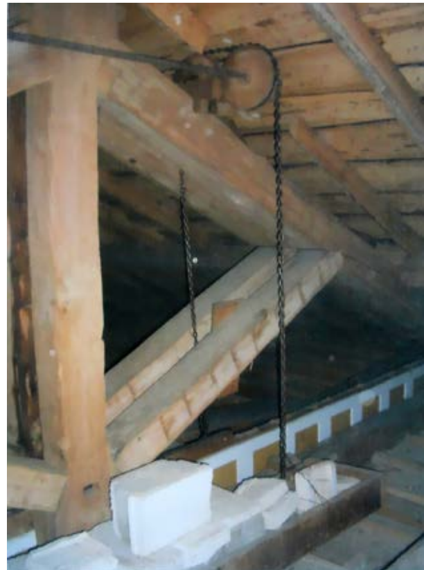
ABOVE: The pulley and chain system used to smoothly raise and lower the meetinghouse partition and counterweight. PHOTO CREDIT: George Webb
